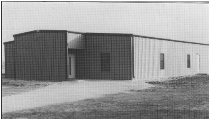
Photo Courtesy Rev. Tommy Tallas Newly constructed Fellowship Building, 1982
