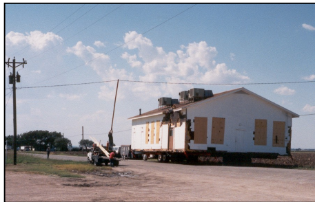
Second Church being moved
