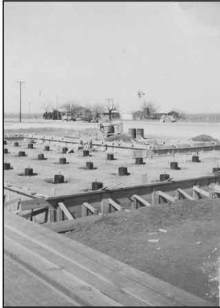
Photo courtesy Ida Chlapek Pier and beam foundation
