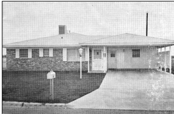
First Parsonage at 113 Norwood in San Angelo
