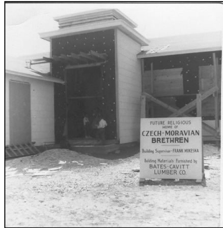
Photo Courtesy Georgia Simcik Construction of second church
